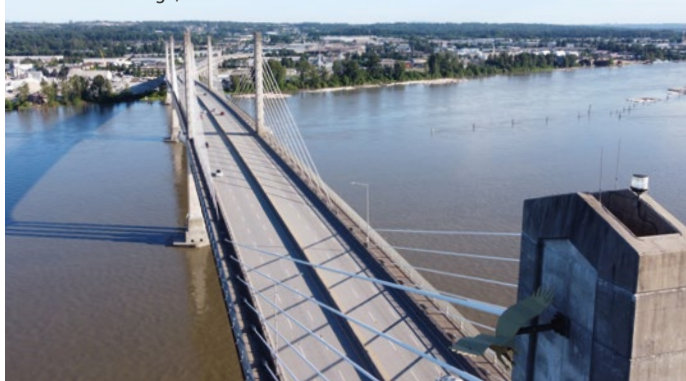
Golden Ears Bridge, Canada
