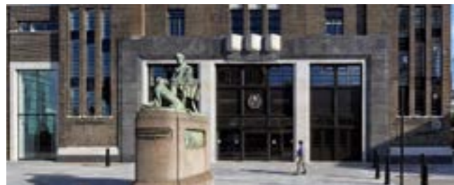
Poplar Affordable Housing & Recreational Centres, UK
