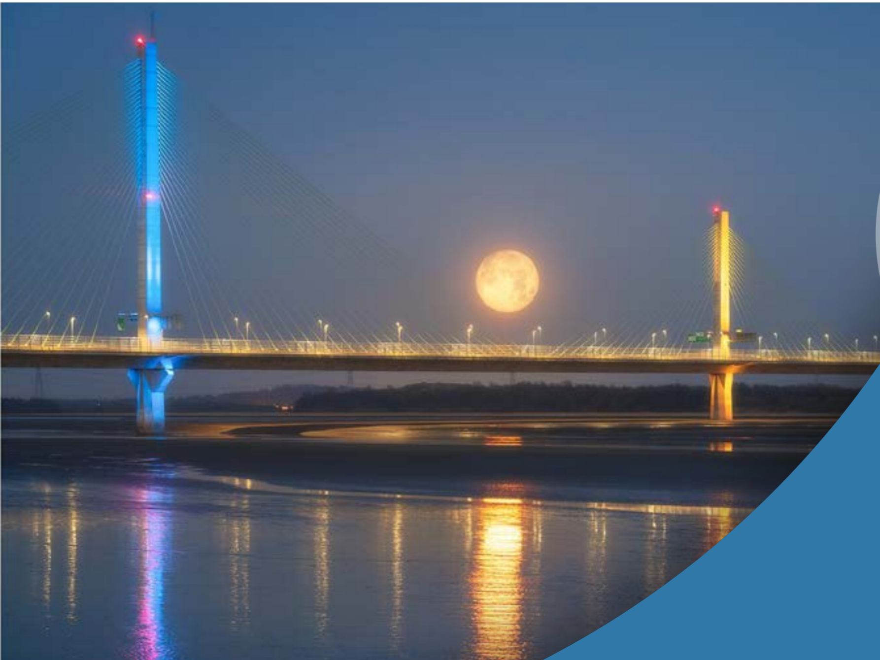
Image: MerseyLink Gateway Bridge, UK (Credit: Andy Light)
