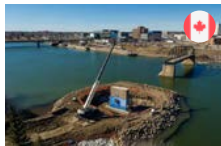
North Commuter Parkway
