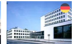
Unna Administration Centre
