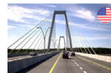
Ohio River Bridges
