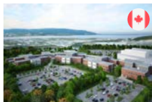
Restigouche Hospital Centre
