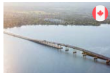
William R. Bennett Bridge
