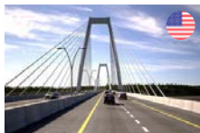
Ohio River Bridges
