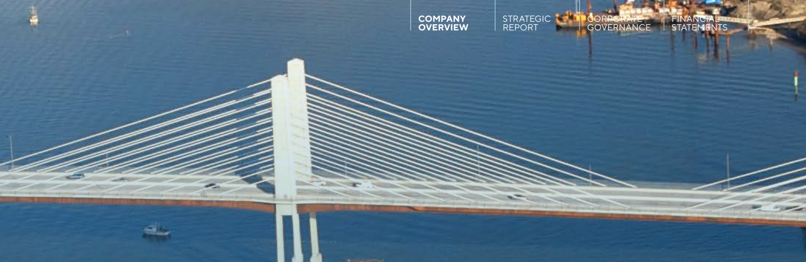
Golden Ears Bridge, Canada
